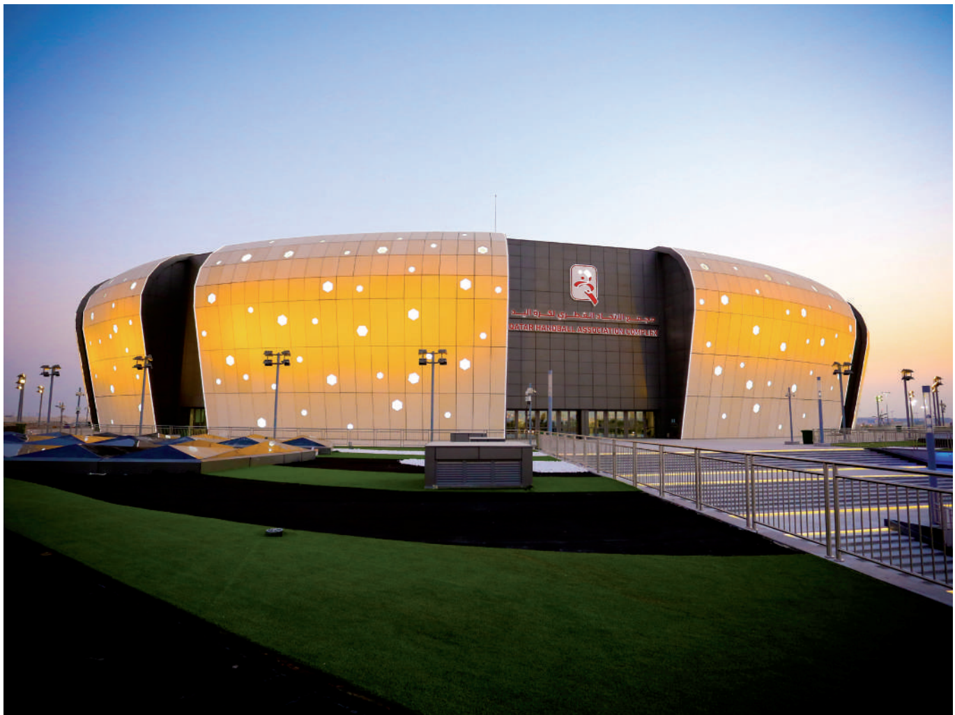
Qatar Handball Association Complex, Doha, Qatar
