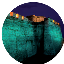
10 Royal Walls of Ceuta Ceuta, SPAIN
