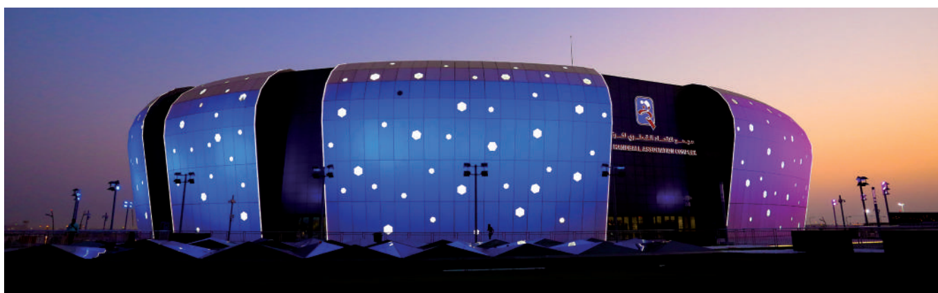
Qatar Handball Association Complex, Doha, QATAR.
